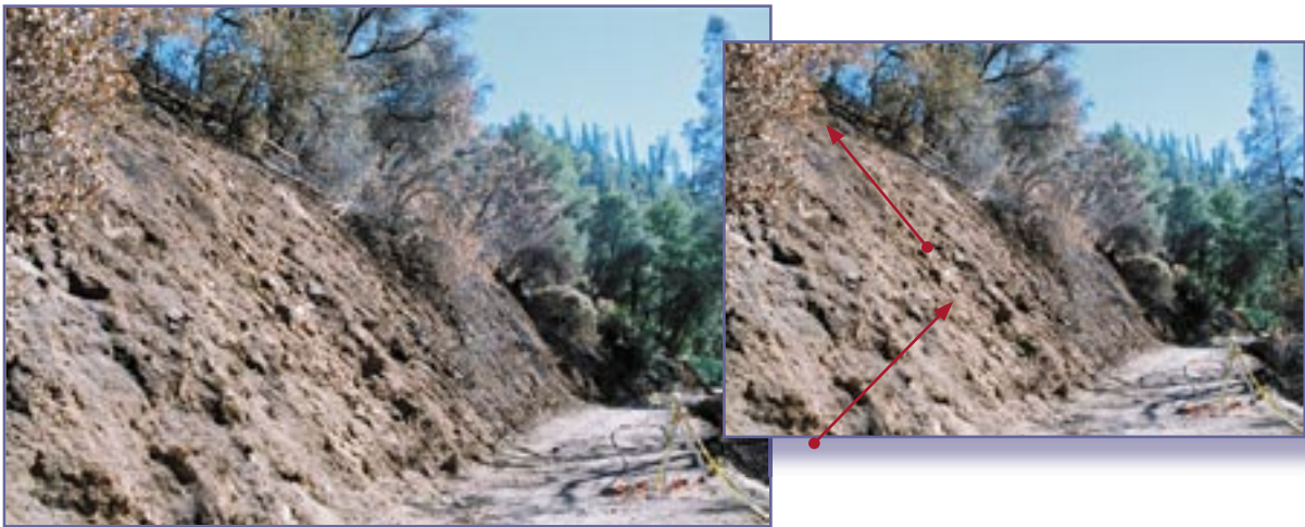
Photo H-14. View from north to south along Lumsden Road above the accident site from next to the top of the line construction and near the reported location where the spot fire was located. Spot fire spread along slope (red arrows) away from camera and then turned up-slope.
